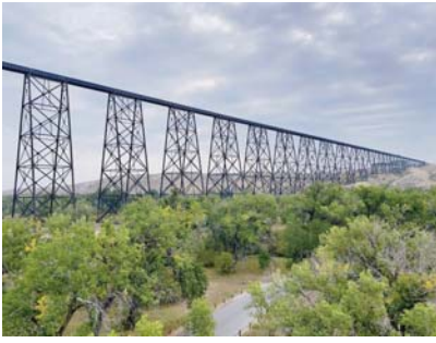
Lethbridge, High Level Bridge
