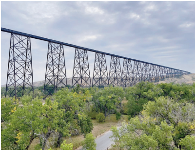
Lethbridge, High Level Bridge
