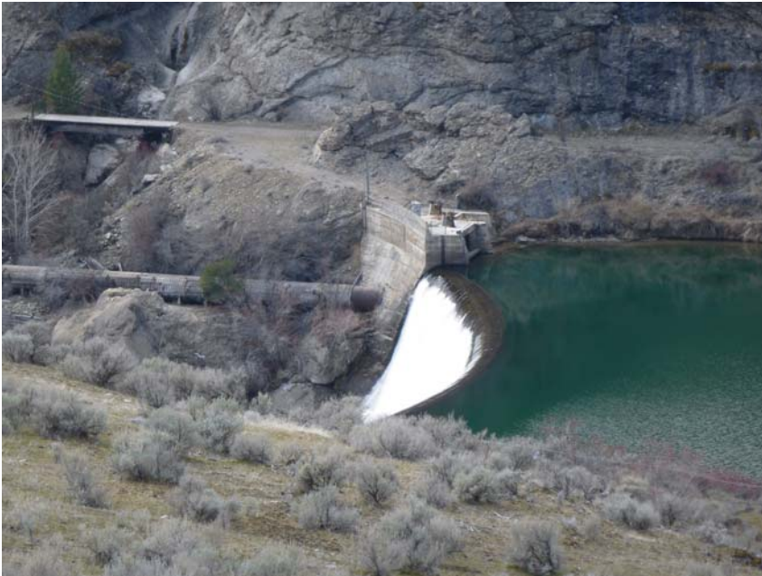
The Enloe Dam
